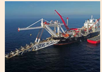
Installation of Nord Stream 2 pipeline Photo: Bernd Wuestneck/dpa (AP)
