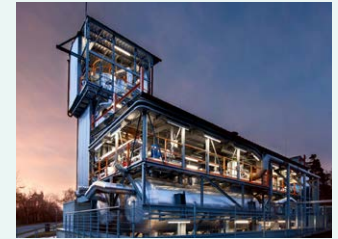
Thermal energy storage TESIS Photo: DLR (CC-BY 3.0)
